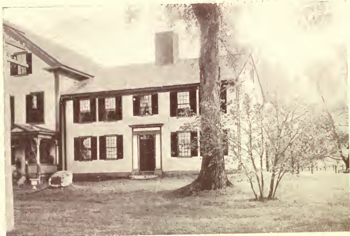
WEBSTER HOUSE AT ELMS FARM
